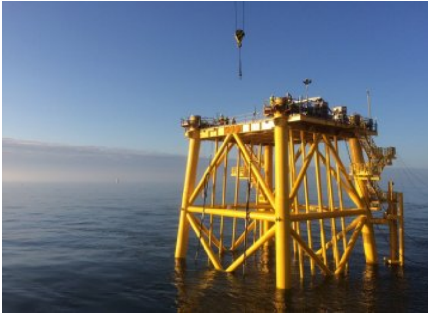
Figure 2-6 Jacket platform example for South Pars Pars 13
