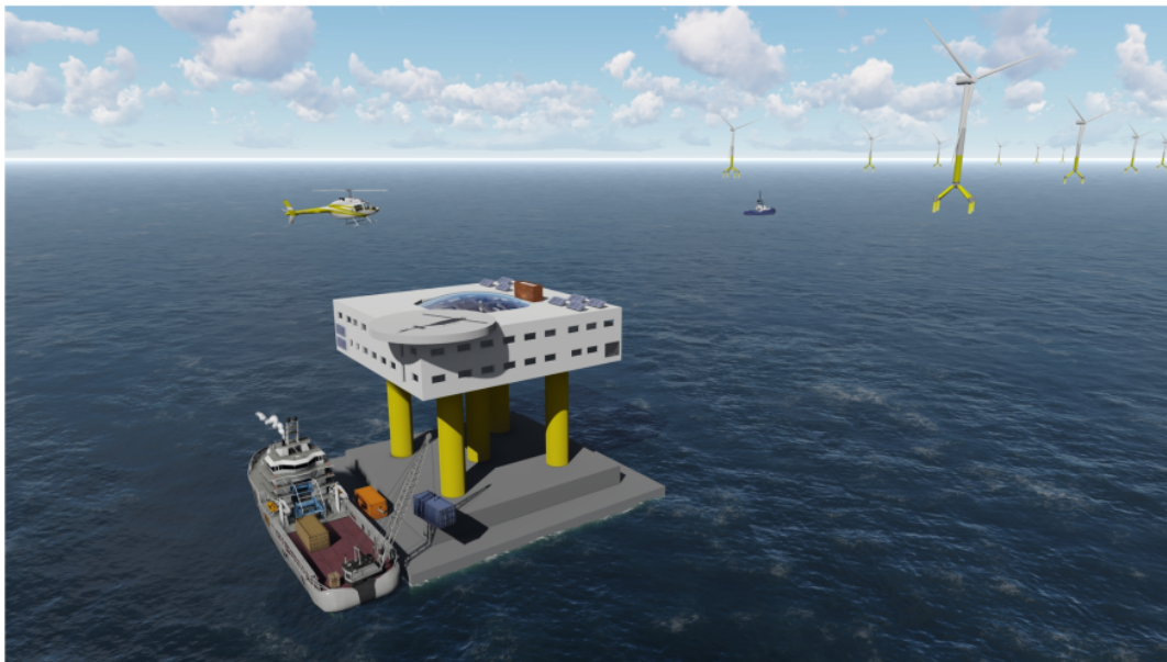
Figure 2.2 Rendering of the Energyhub@Sea purposed for the North Sea (Mediterranean build is without columns, LWET/GICON)
